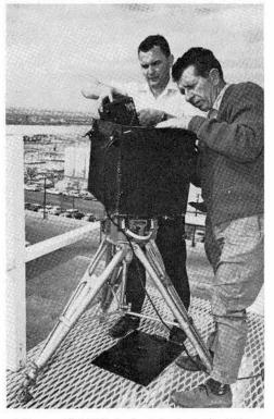
70-mm CAMERA is installed at the Albuquerque Sunport by Clarence Robertson, left, and John Banker (both 7226). The camera will be used in a joint city and county study of air pollution. It will make photogarphs every five minutes.
